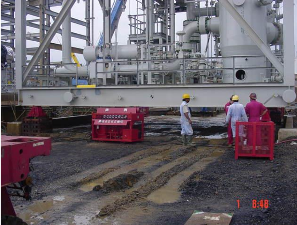
JACKING DOWN HAS BEGUN
