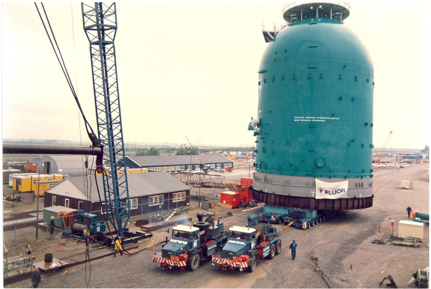
TWO, 3 METER WIDE, 16 AXLE TRAILERS HAULING A 600 Te REFINERY VESSEL
