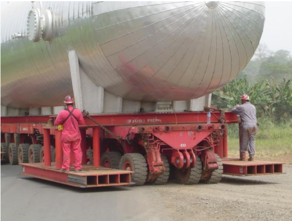
LOAD SPREADERS AND PIPE STANCHIONS CONNECTED TO THE STAGING BEAMS
