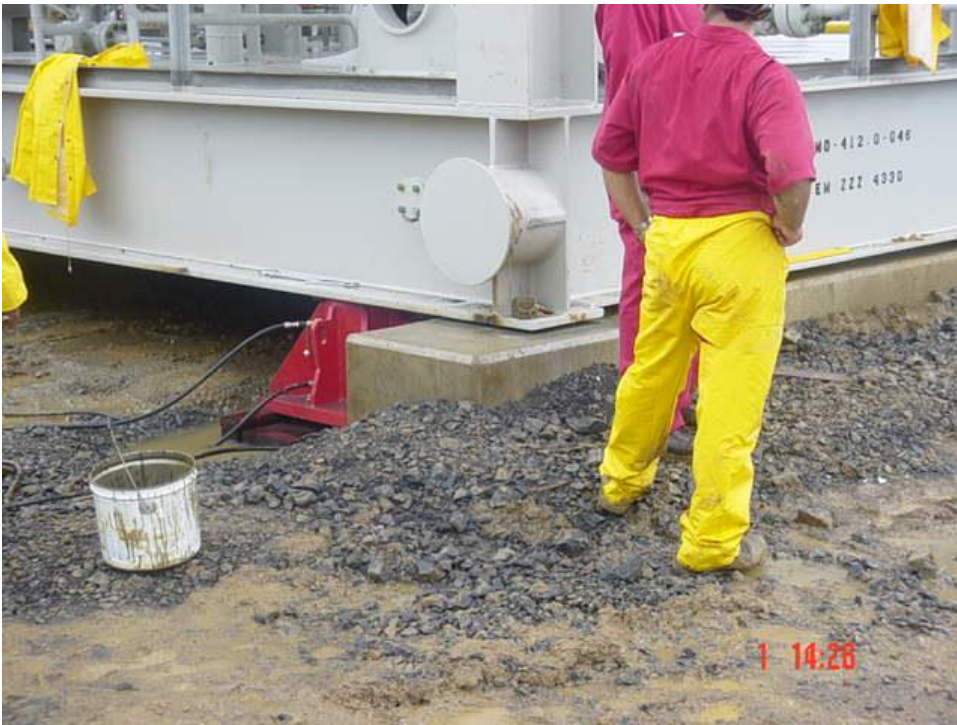
THE MODULE DOWN ON THE FOUNDATION
