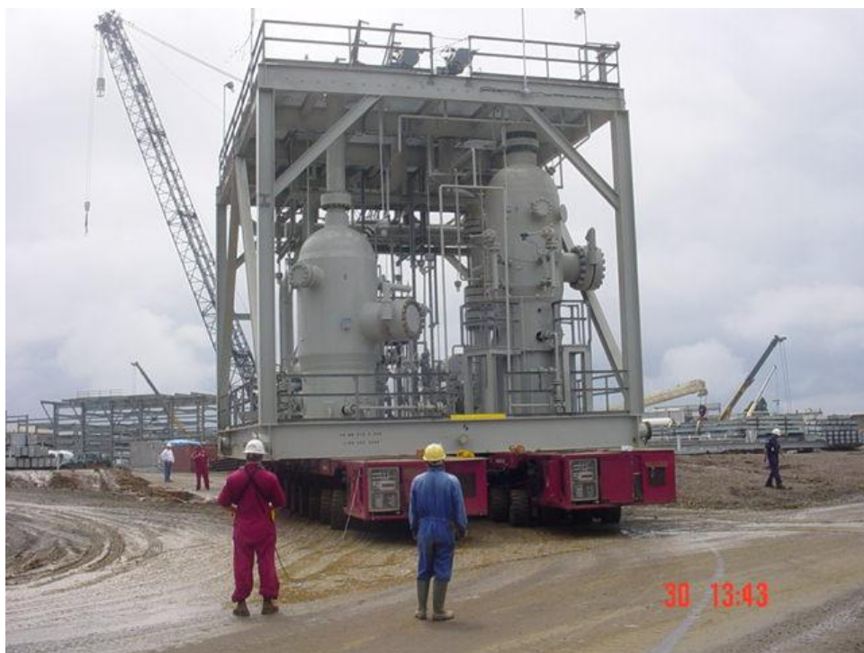
EQUIPMENT MODULE ARRIVING AT SITE
