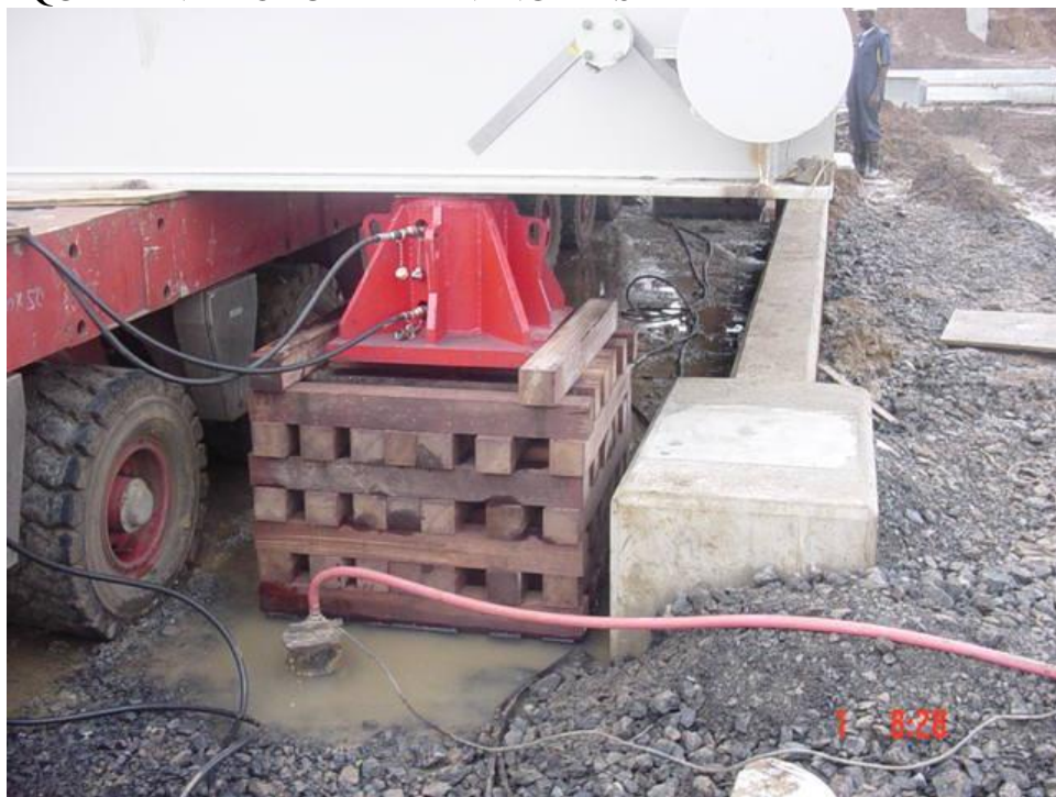
CRIBBING AND CLIMBING JACKS IN PLACE
